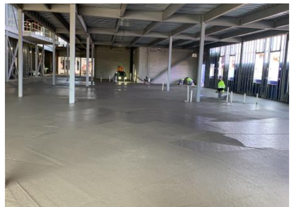
SOG in the future art labs getting poured (09/29/2022)
