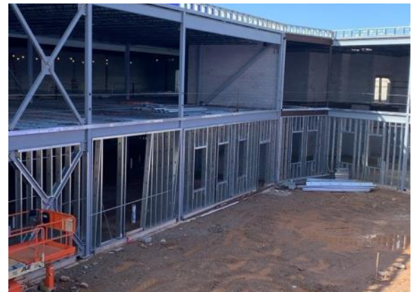
East courtyard exterior steel stud framing (09/21/2022)
