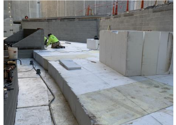
Auditorium stepped seating structure gets set in place (09/27/2022)
