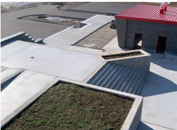
Completed grandstand stairs and ADA ramp (09/21/2022)
